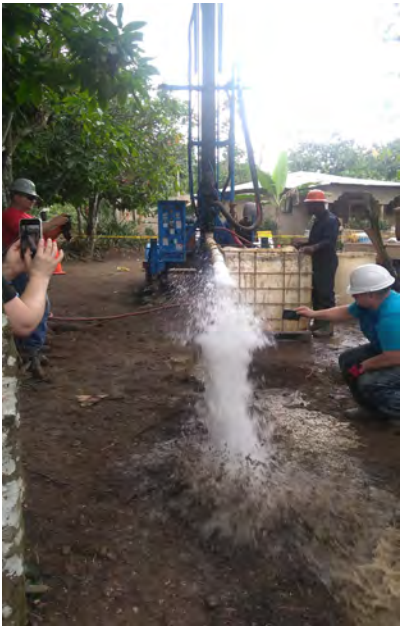
The team flushes the borehole for the well.
